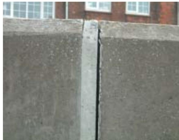
**Figure 4.4 Close of damaged joints in crest wall**
